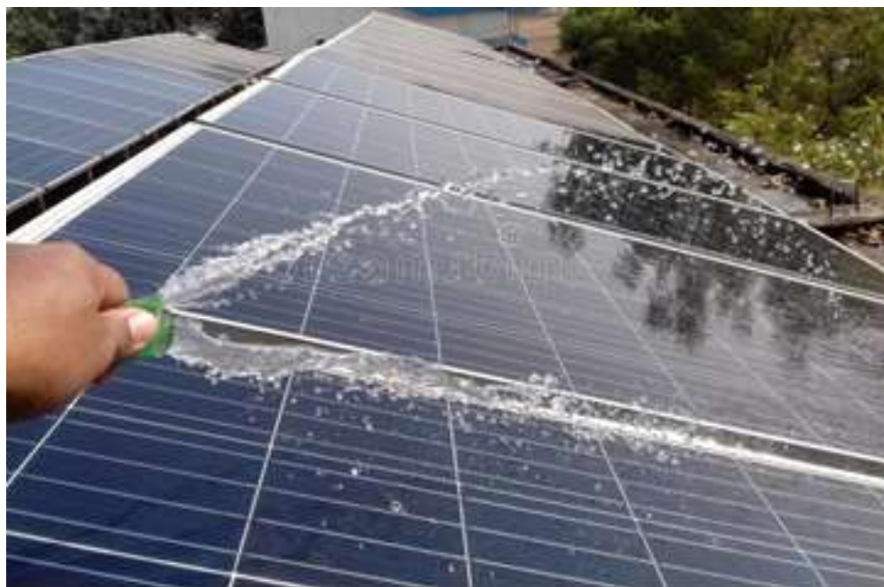
Figure 3: Cleaning of Solar PV Module for better absorption of solar radiation
